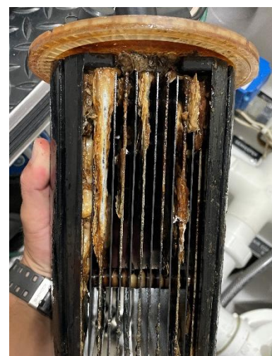
Calcium scale is often the first indication of the ClearCell Electrode nearing the end of its life expectancy.
